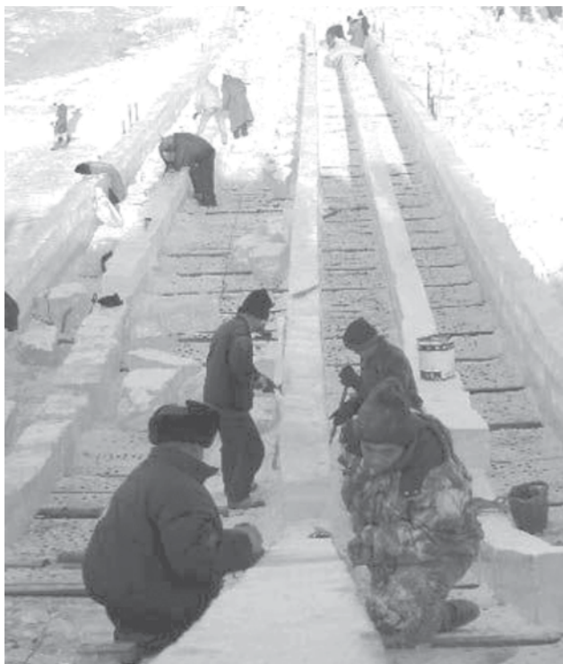
An ice slide is built by workers in Harbin, northeast China's Heilongjiang Province, on 15 Dec, 2006. More than 100 meters long and 15 meters high, the ice slide will be completed in late December.—XINHUA
