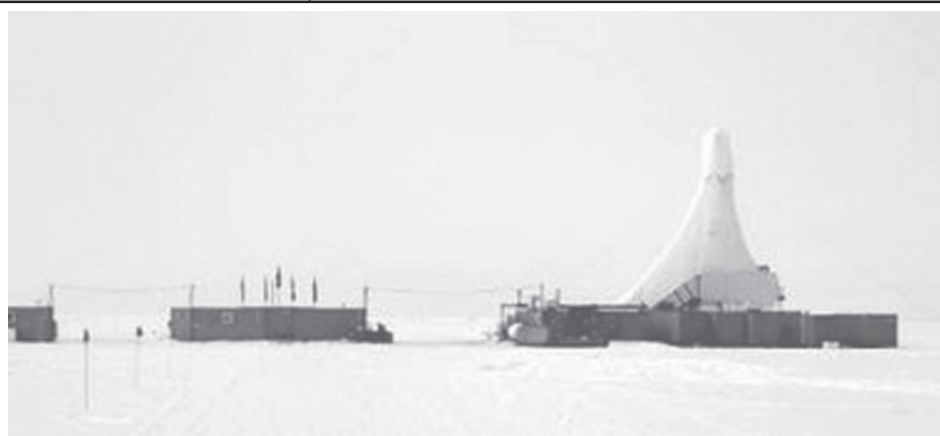
The ANDRILL site is seen on the Ross Ice Shelf in Antarctica on 12 Dec, 2006. The project, short for Antarctic geological drilling, aims to drill back in time to about 10 million years ago for possible clues to the consequences of global climate change. The drill rig is covered in a white tent to keep temperatures about 50 degrees F (10 degrees C) so that the drill's hydraulics can work.—INTERNET
