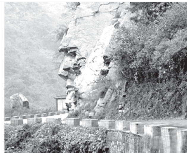
The photo taken on 26 Nov, 2006 shows a profile of human face at turning point of a mountain road in Shiquan county, Shaanxi Province. The profile was cut accidentally by road constructors in 2001.—XINHUA
