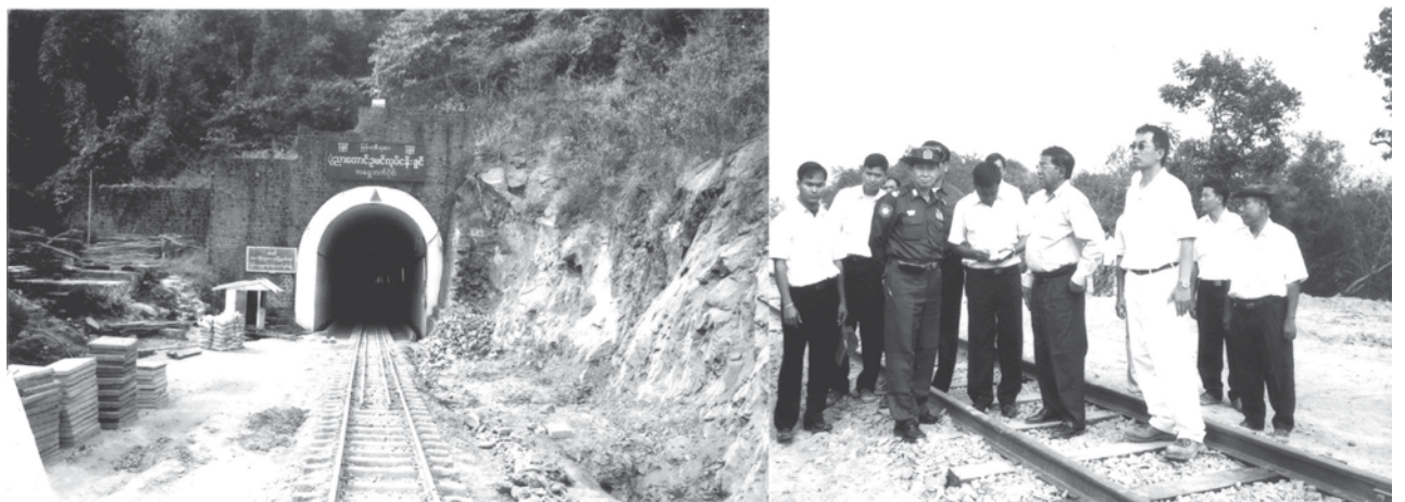
Minister for Rail Transportation Maj-Gen Aung Min looks into progress in building of Ponnyataung Tunnel in Gangaw Township. —MNA
