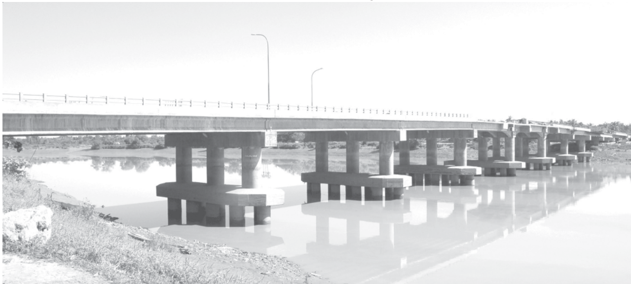
Ngamoeyeik Bridge (Kamakyi) construction is in progress. — MNA
