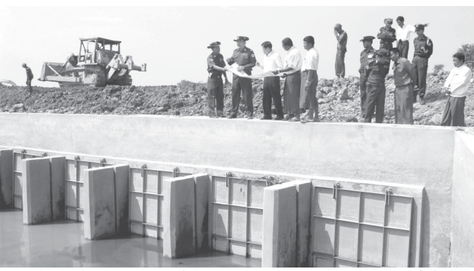
Commander Brig-Gen Hla Htay Win inspects construction of sluice gate on embankment to Bago River. — YANGON COMMAND
