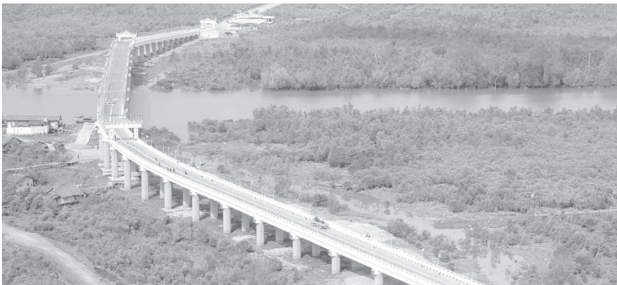
Minkyaung Bridge on Yangon-Kyaukpyu Highway helps cement national strength and unity.
