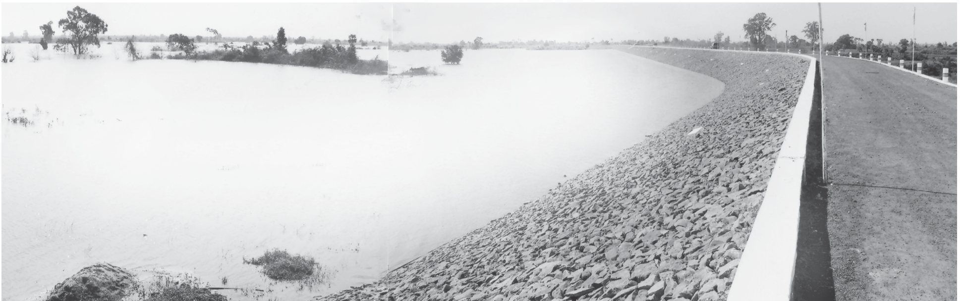
Paygyi Dam built in Kanbalu Township, Shwebo District, Sagaing Division. — A&I
