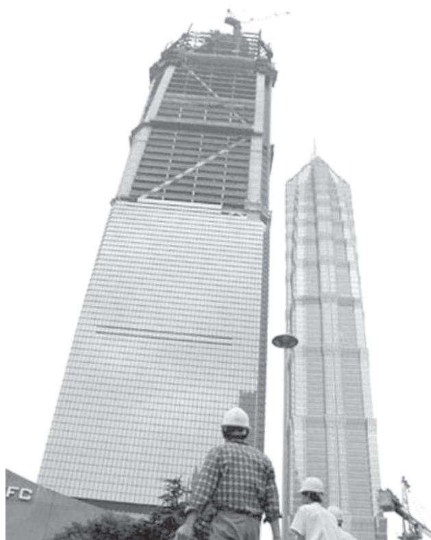
The Shanghai World Financial Centre, is seen under construction near Jin Mao Tower, China’s tallest building, in Shanghai’s Lu Jia Zui financial district on 24 Oct, 2006. —XINHUA
