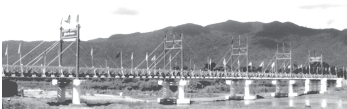
Phainglin Bridge in Tamu Township, Sagaing Division. — CONSTRUCTION
