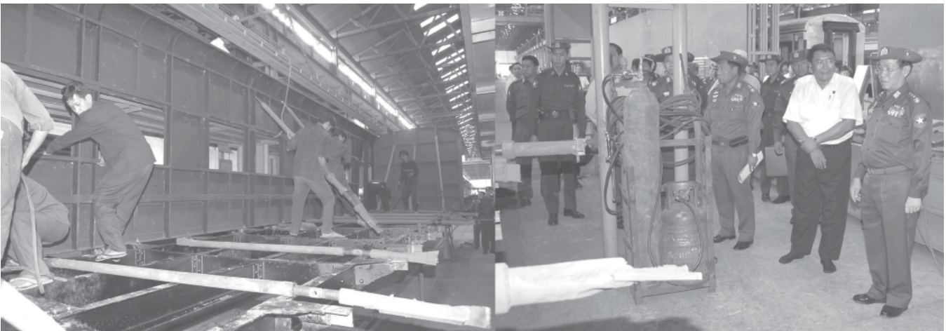
Prime Minister General Soe Win inspects construction of carriages at Myitnge Carriage and Wagon Shed. — MNA
