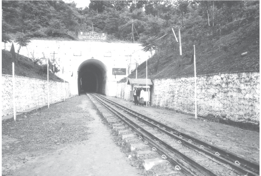
Ponnyataung Railroad Tunnel Construction Project.
