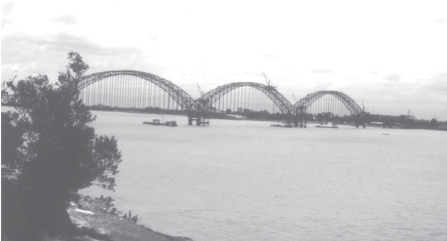
Progress of Ayeyawady Bridge (Yadanabon) construction project seen from Sagaing bank.
