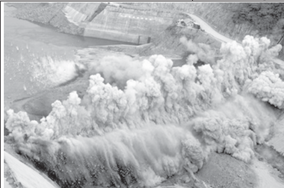
In this photo released by China's Xinhua News Agency, cofferdam of the Longtan hydropower station, located on the upper reaches of the Pearl River in southwest China's Guangxi Zhuang Autonomous Region, is seen being demolished for the safety of the dam during flood season, on 20 Sept, 2006.—INTERNET
