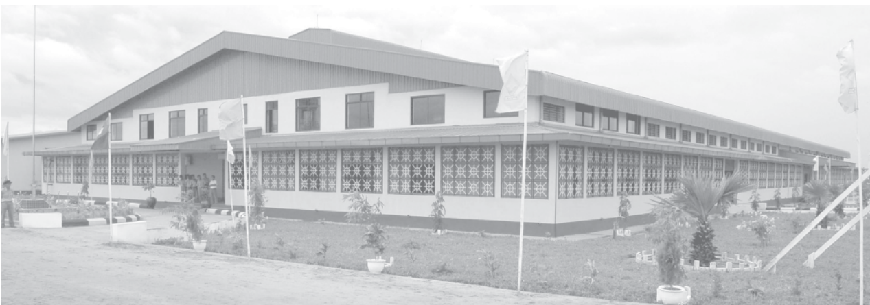
Garment Factory (Pakokku): The factory is 340 feet long, 150 feet wide and 20 feet high. It is a reinforced concrete building. The factory is equipped with one 11-KV sub-power station, a water tank, warehouses and 704 machines including 526 multi-functional sewing machines. A total of 816 employees have been appointed at the factory. The strength of the workforce is 31 officers and 1,597 staff members. The factory will manufacture 1.2 million pieces of garment yearly.
