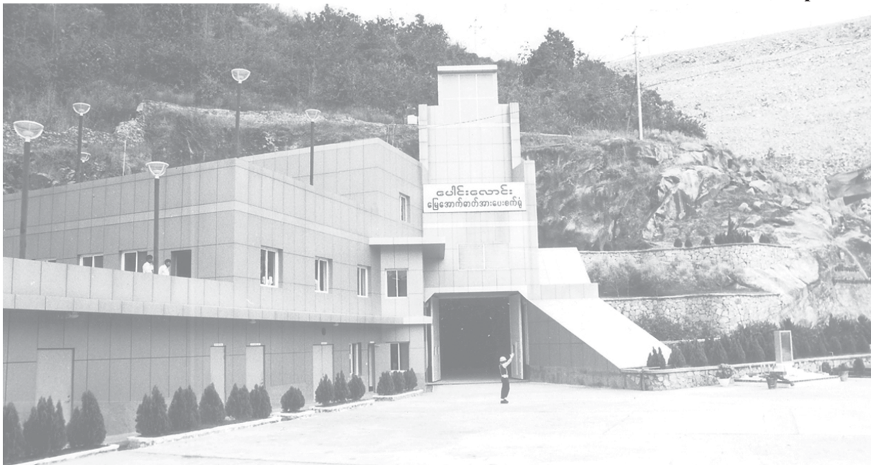
Paunglaung underground power station in Pyinmana Township.
