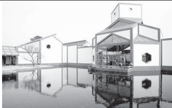
The photo taken on 19 Sept, 2006 shows the view of the newly-designed Suzhou Museum in Suzhou, a scenic city in east China’s Jiangsu Province, 19 Sept, 2006. Designed by noted Chinese-American architect Ieoh Ming Pei, the museum will be opened to the public in the Mid-Autumn Festival, which falls on 6 Oct this year.—INTERNET
