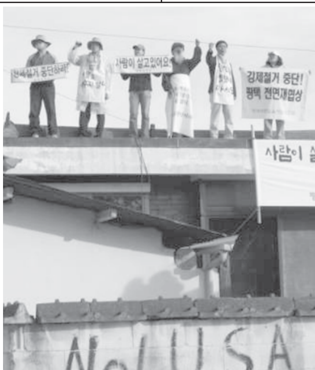
Protesters shout slogans on the roof of a house as they try to stop its demolition to make way for a US base extension in Pyongtaek, about 70 km (44 miles) south of Seoul, on 13 Sept, 2006. South Korea's Defence Ministry began demolishing empty houses to make way for the extension of the US base site in the township. The slogans reads "Stop removal of house, People live in here."—INTERNET
