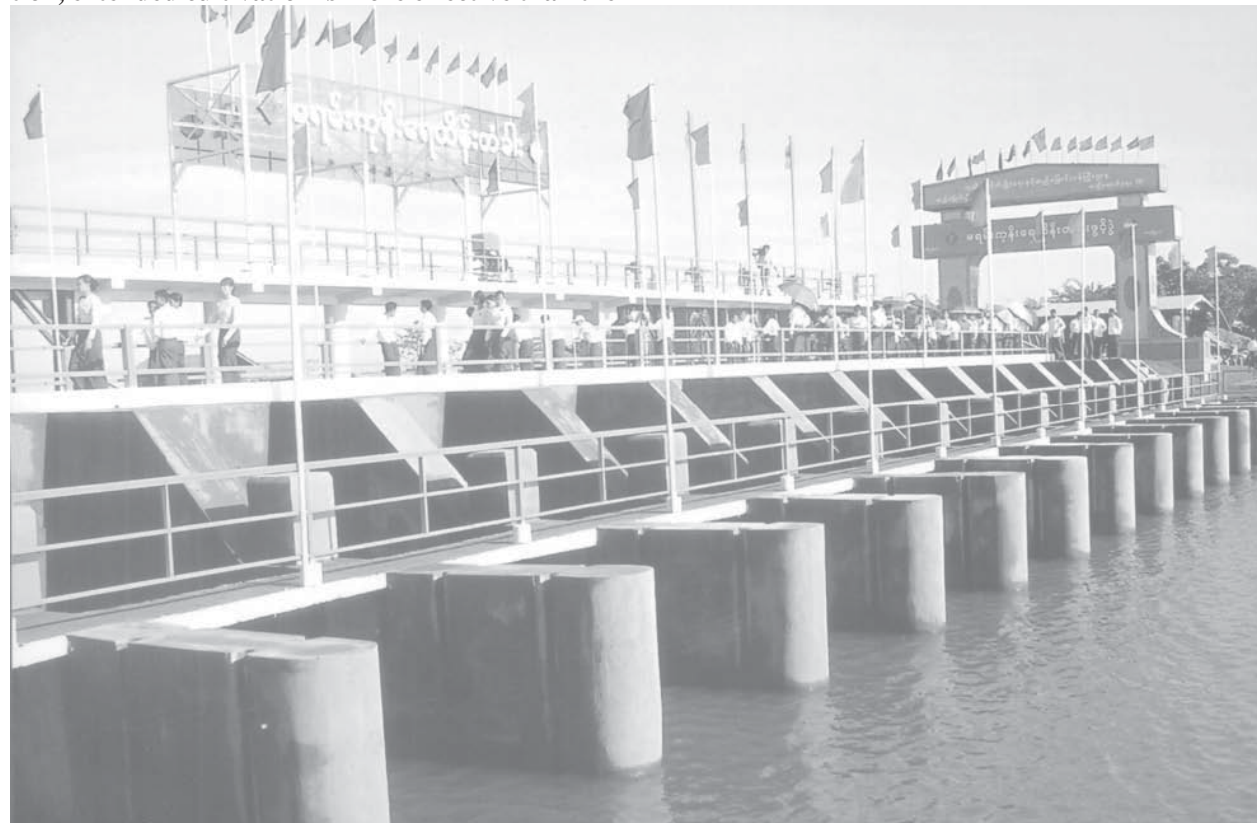
Mayangon Sluice Gate in Thaton Township.
