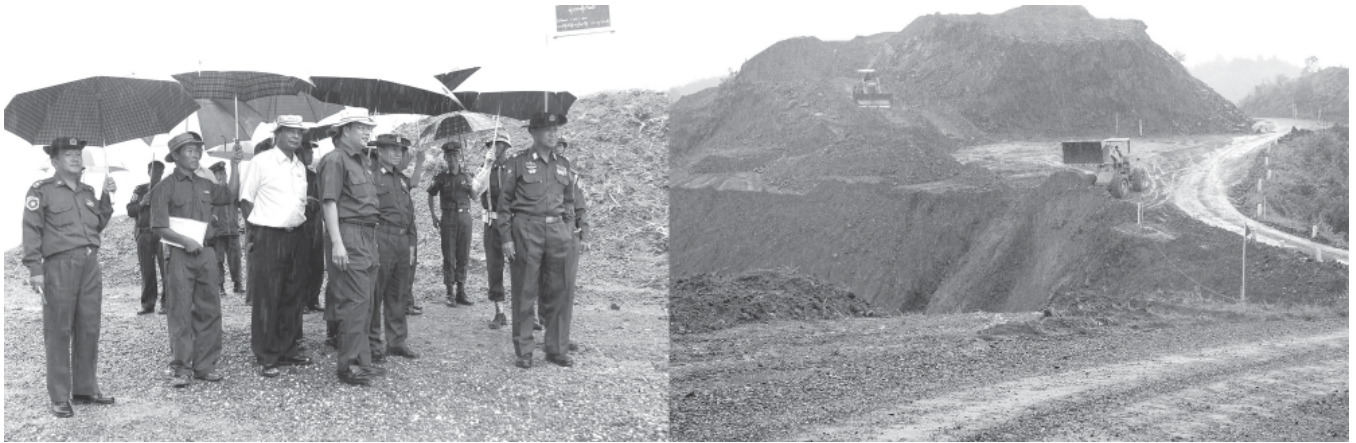
Lt-Gen Khin Maung Than inspects repair work on Minbu-An Road. — MNA
