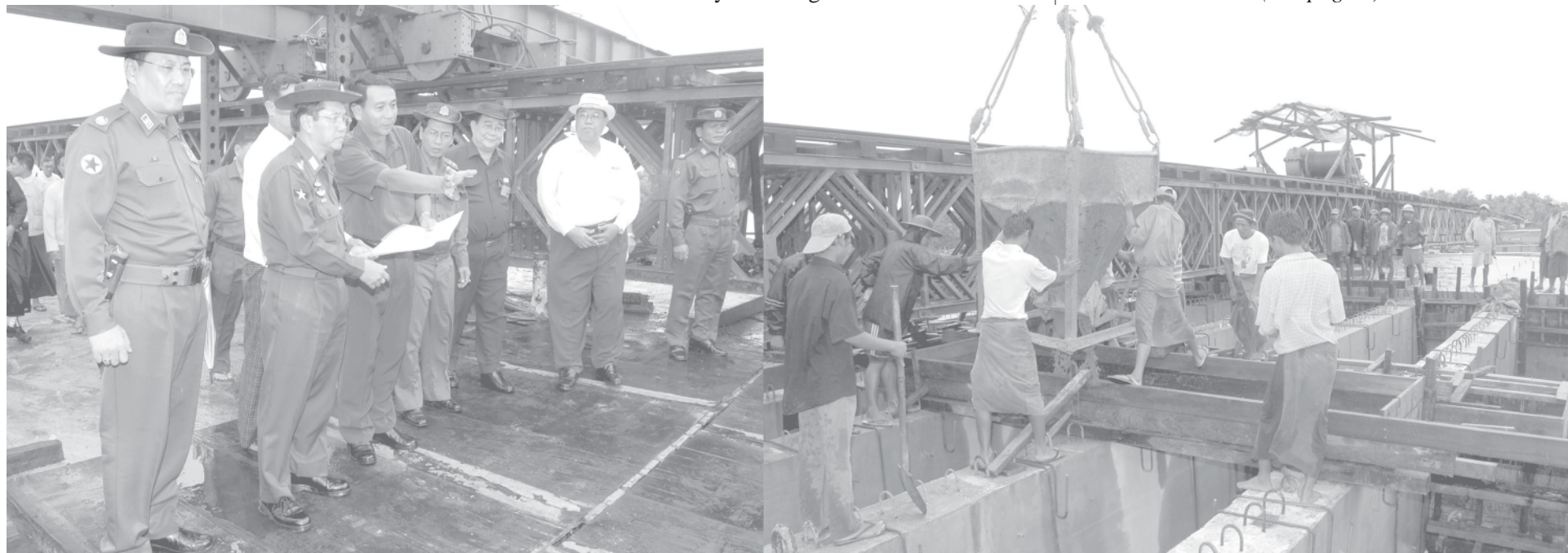
Lt-Gen Myint Swe inspects construction of Ngamoeyeik Bridge (Kamakyi). — MNA
