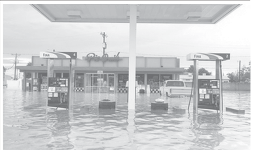
A convenience store in downtown Hatch, New Mexico, is seen after a monsoon storm caused flooding in the town on earlier 15 Aug, 2006.—INTERNET
