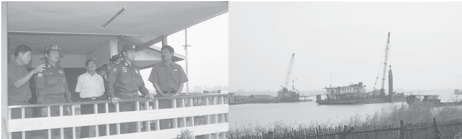
Lt-Gen Khin Maung Than inspects construction of Ngawun Bridge (Myokwin). — MNA
