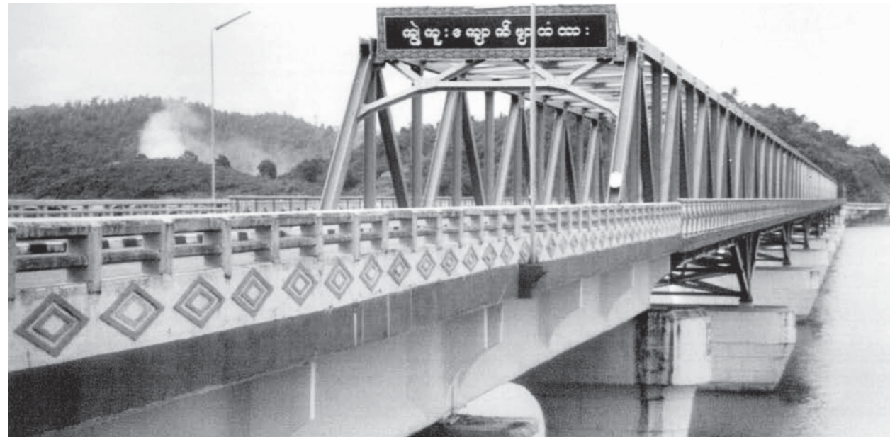
Kywegu-Kyaukphya Bridge near Myeik.
