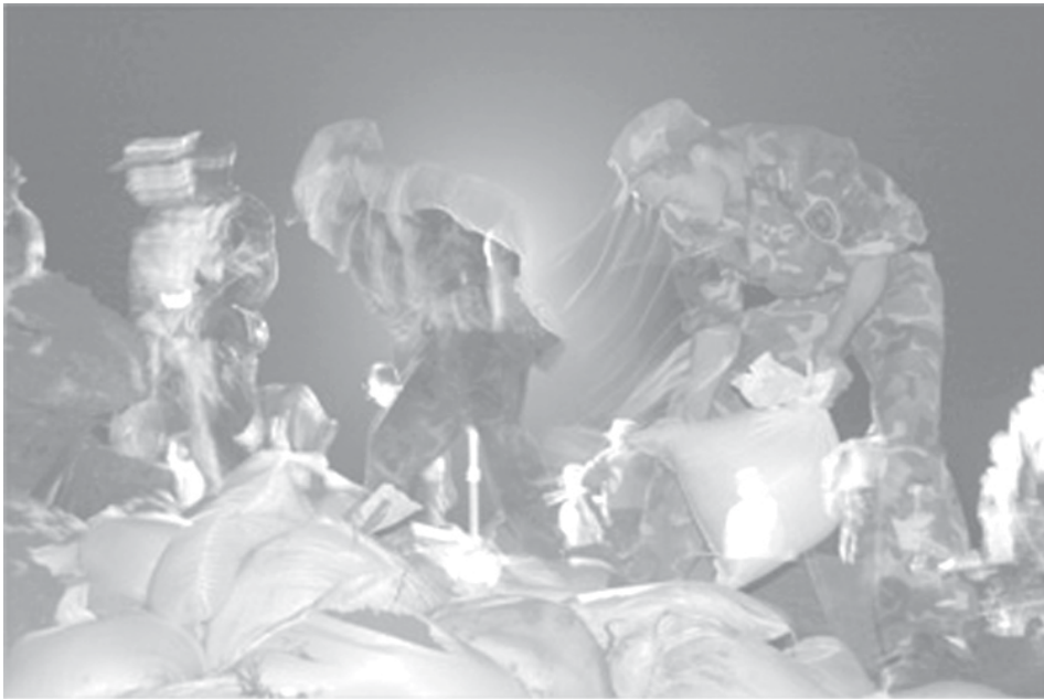
Soldiers pile sandbags up to reinforce the bank of Sankeng River in Qingyuan, southeast China's Guangdong Province, on 4 Aug, 2006.—INTERNET
