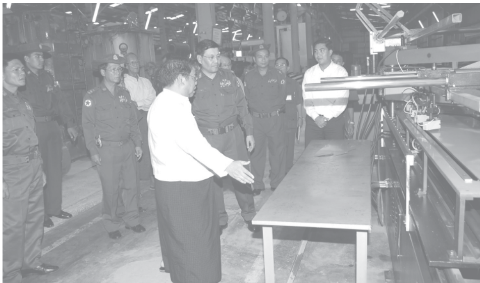
Commander Brig-Gen Hla Htay Win inspects Transformer Factory of Soe Electric and Machinery Co Ltd in Industrial Zone in Dagon Myothit (South). — MNA
