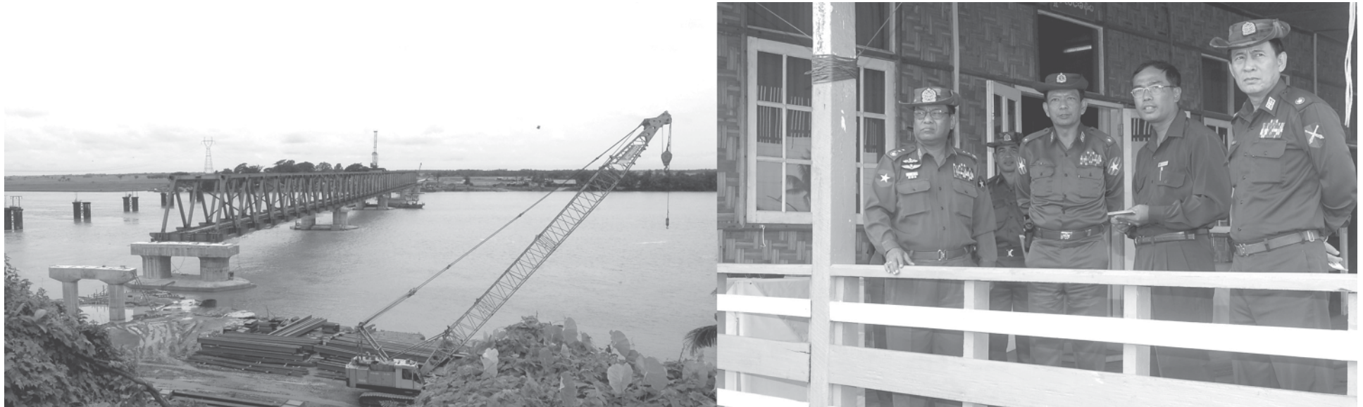
Lt-Gen Maung Bo inspects construction of Sittoung Bridge (Moppalin). — MNA
