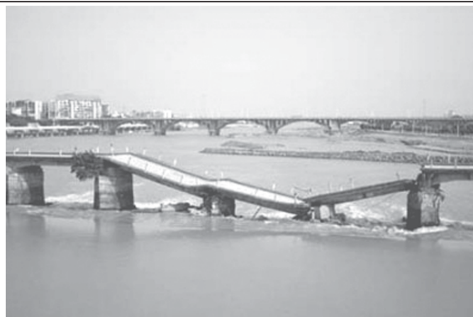
The picture shows a collapsed bridge in Quanzhou, East China's Fujian Province, on 23 July, 2006. The tropical storm Bilis and floods might cause the collapse of the Shunji Bridge, built in 1211 during the Southern Song dynasty (1127-1279), sources said. —INTERNET
