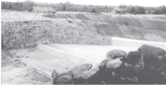
The spillway of the Hlaingchaung Dam.
