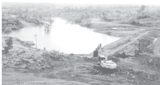
The North Yama supporting dam project is nearing completion.
