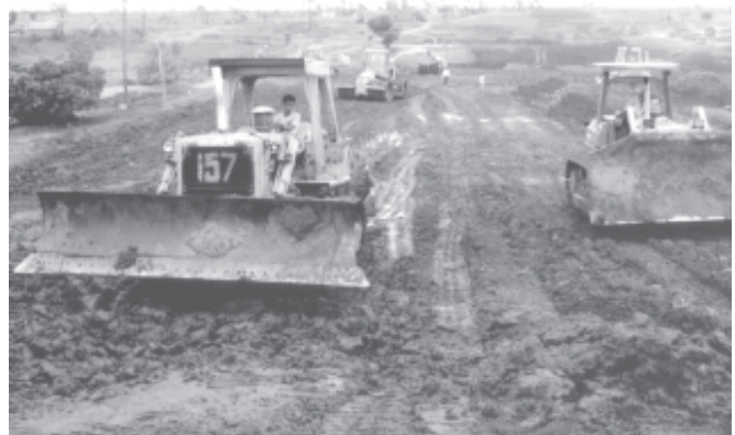
Heavy machinery operating to prepare land at the Hlaingchaung Dam Project.
