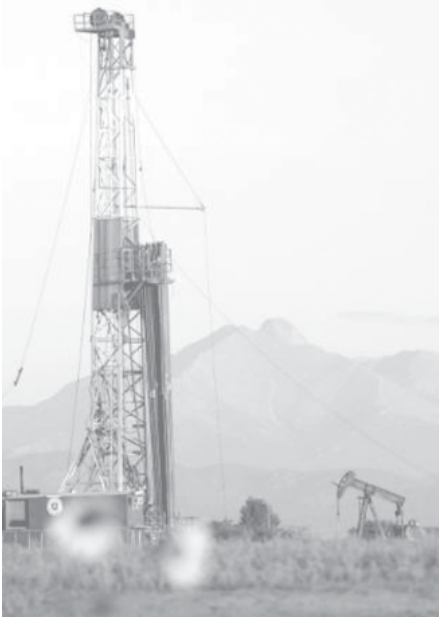
A new oil well is drilled near Dacono, Colorado on 12 July, 2006. The Denver-Julesburg basin oil field near Denver stretches from Wyoming. —INTERNET
