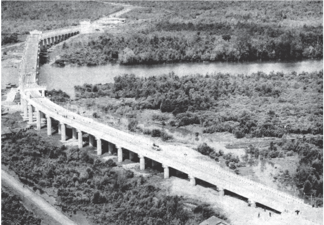
Yangon-Kyaukpuy highway and Minkyaung bridge on it were put into service on the same day.
