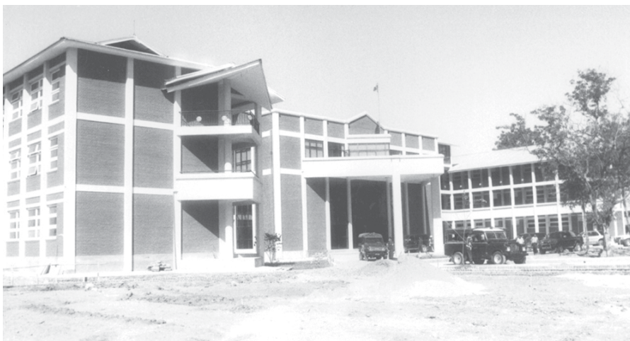
The three-storey building of Pyay University in Bago Division (West).
