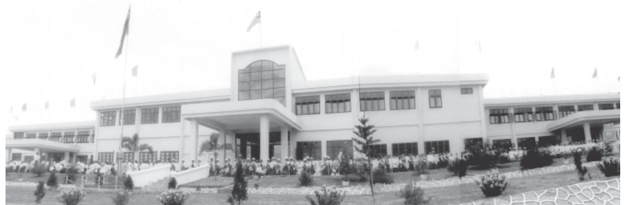
200-bed General Hospital in Kengtung, Shan State (East).
