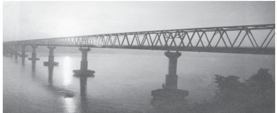
Ayeyawady river crossing Nawaday Bridge, which is 4,183 feet long, in Pyay, Bago Division.
