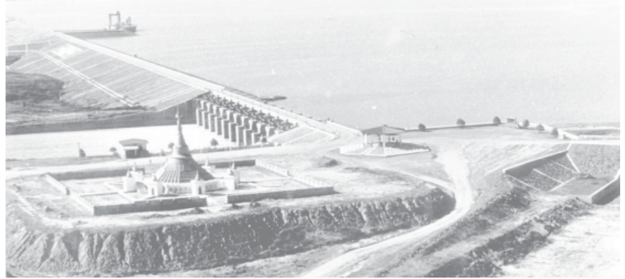
Thaphanseik Dam in Kyunhla Township, Sagaing Division can irrigate 500,000 acres of farmland and generate 117.2 million kilowatt hours of electricity a year. It is the largest of its kind in Myanmar.
