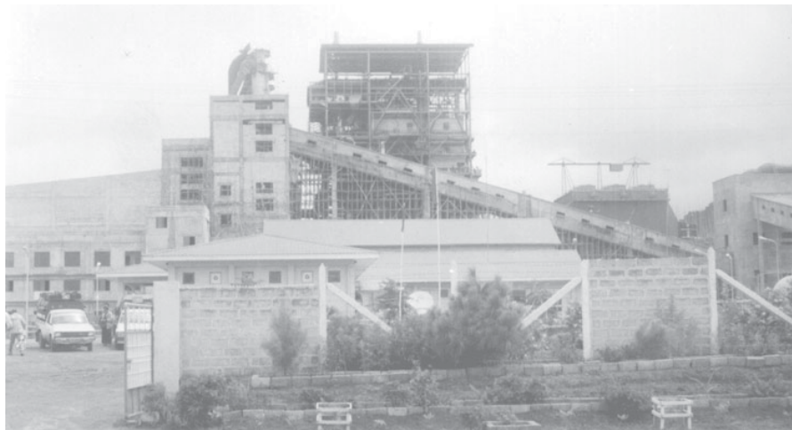
Coal-fired power station being run in Tikyit Region in Shan State (South).
