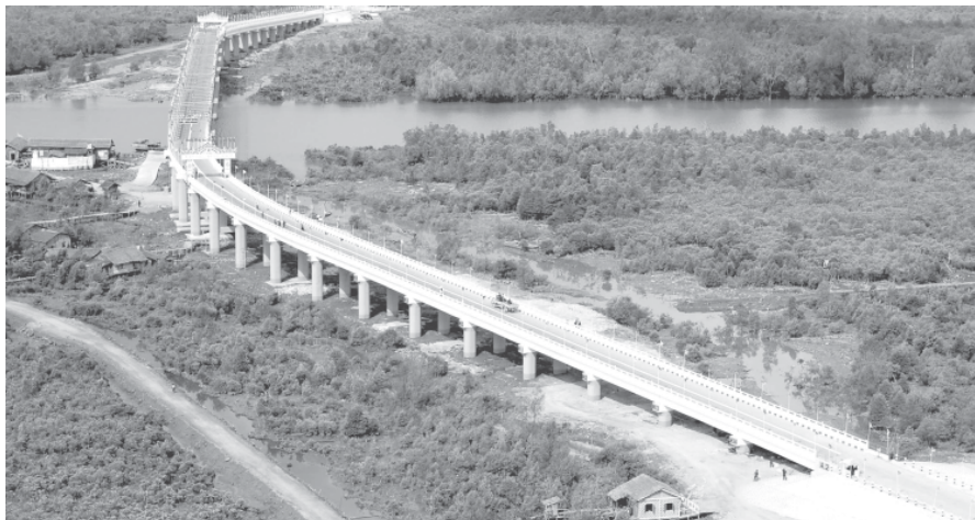
With the length of 2,704.2 feet, Minkyaung Creek Bridge in Rakhine State is the longest one among the 13 completed major bridges built on Taungup-Kyaukpyu road section in Rakhine State in the time of the Tatmadaw Government.
