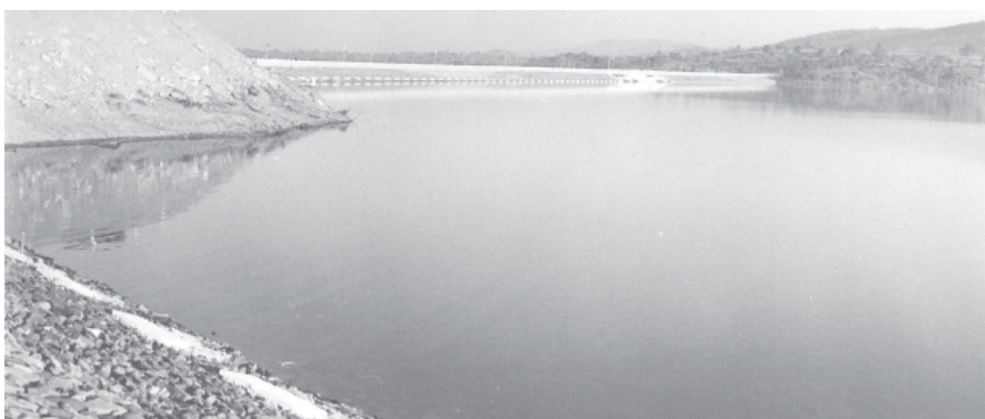
Newly-inaugurated Yagyi Dam in Kyaukpadaung Township, Mandalay Division.
