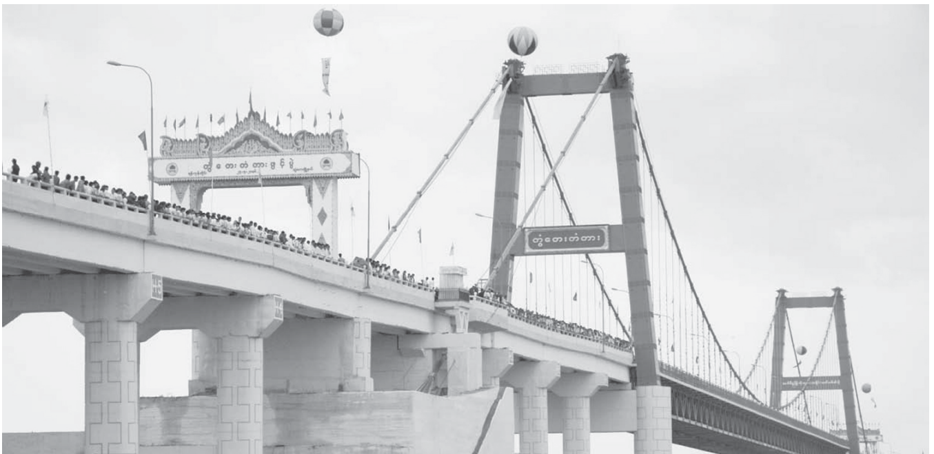
Twantay Bridge across the Twantay Canal near Phaya Ngokto Village in Twantay Township, Yangon South District is 3,570 feet long .
