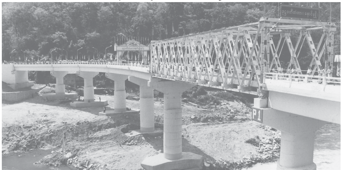
Dokhtawady Bridge (Nawngkhio) linking Yaksauk Township in Shan State (South) and Nawngkhio Township in Shan State (North).
