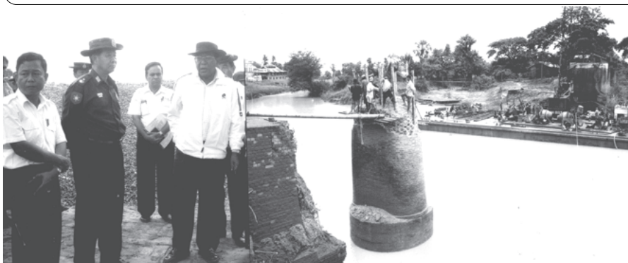
Maj-Gen Aung Min inspects construction of Hparshin Creek Bridge. — MR
