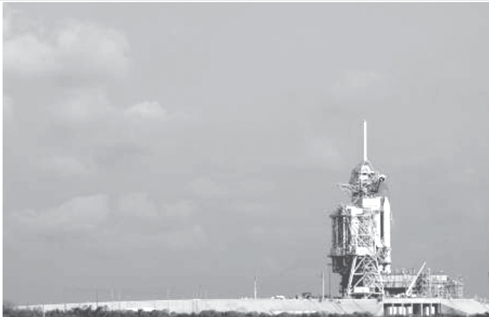
The Space Shuttle Discovery sits on its launch pad while being prepared for Mission STS-121 in Cape Canaveral, Florida, on 30 June, 2006. The shuttle is covered by the protective Rotating Service Structure. —INTERNET
