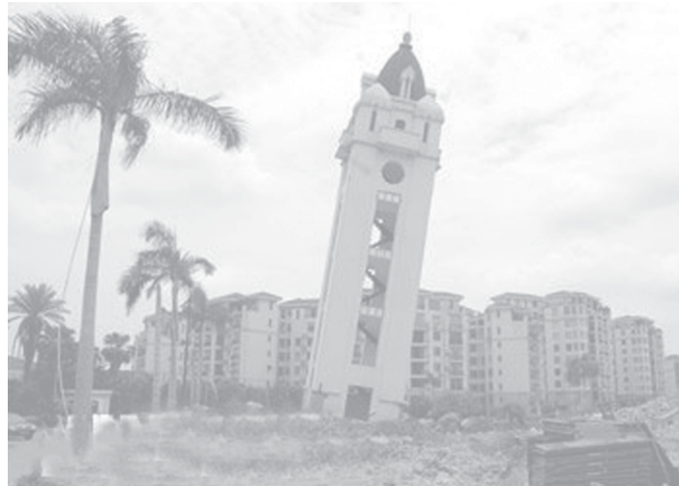
A leaned bell tower is seen at a residential area in Liuzhou, south China's Guangxi Zhuang Autonomous Region, on 27 June, 2006. The demolition of the tower earlier failed and made it leaned. —INTERNET
