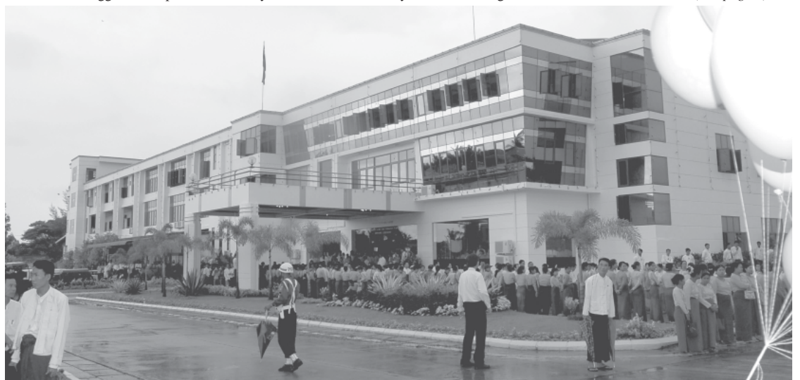
Newly opened Yuzana Palm Oil Refinery and Dry Fractionation Plant in Shukhintha Ward in Thakayta Township. — MNA
