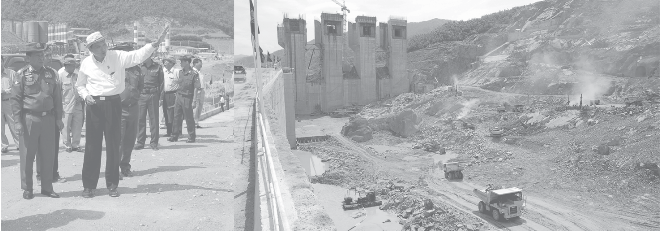
Lt-Gen Ye Myint inspects Yeywa Hydrel Power Project site. — MNA
