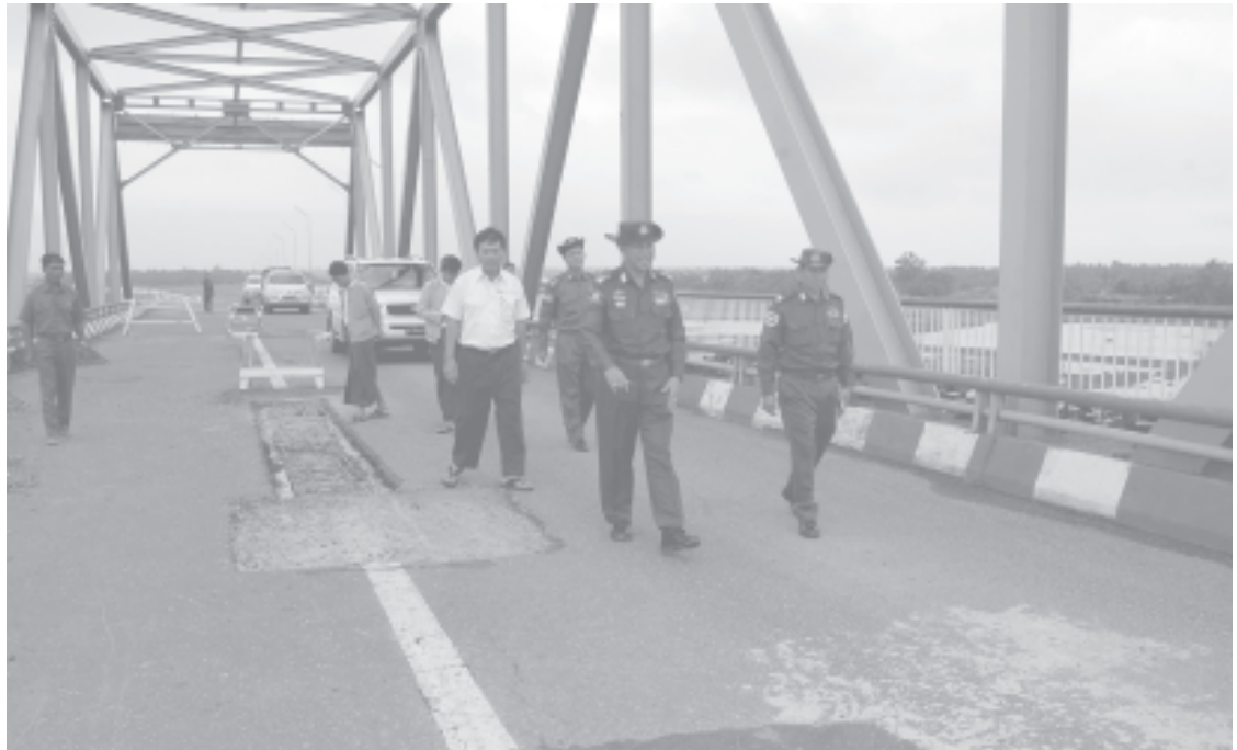
Lt-Gen Khin Maung Than inspects Minchaung Bridge on Yangon-Sittway Highway. —MNA
