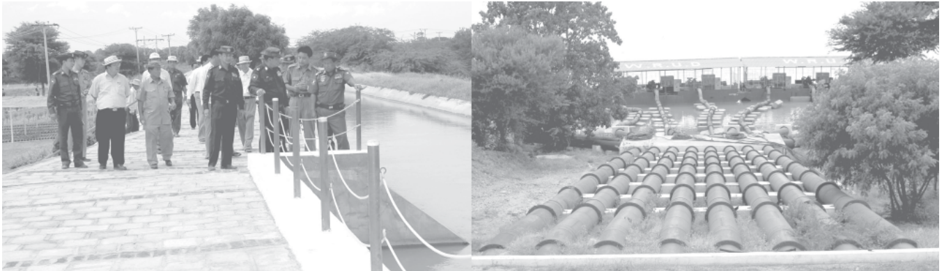
Lt-Gen Ye Myint of Ministry of Defence inspects water supply facilities of Lawkananda River Water Pumping Station. — MNA
