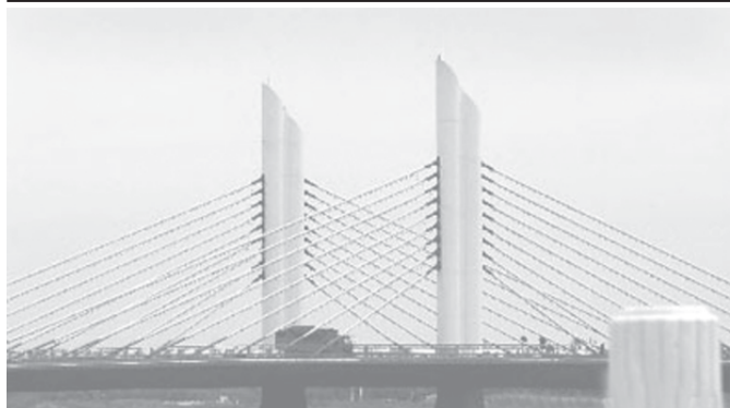
The cable-stayed bridge over the Aiyi River in Yinchuan, capital city of Ningxia Hui autonomous region completed safety tests recently. Being the widest single amplitude cable-stayed bridge in the world, it is 206 metres long, 60 metres wide and 8.8 metres high.—INTERNET
