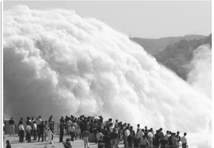
Residents look at water gushing out from the Xiaolangdi Reservoir into the Yellow River in China's Henan Province, on 15 June, 2006. About 3,000 cubic metres of water will gush out of the reservoir per second in the next 15-20 days to wash the sands in the river into the sea, China Daily reported. —INTERNET
