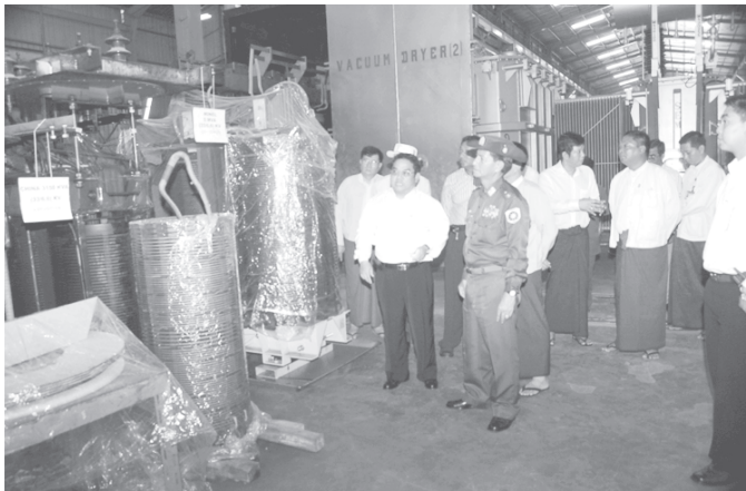
Minister Maj-Gen Khin Maung Myint inspects transformer factory in Dagon Myothit (South) Township. — MNA
