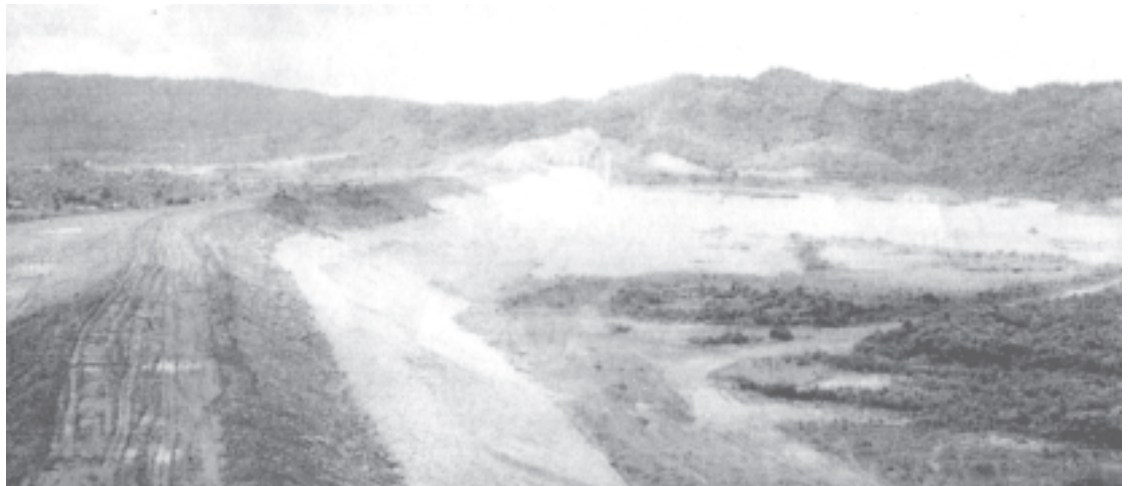
Kataik Dam under construction in Paung Township, Mon State. — MNA
