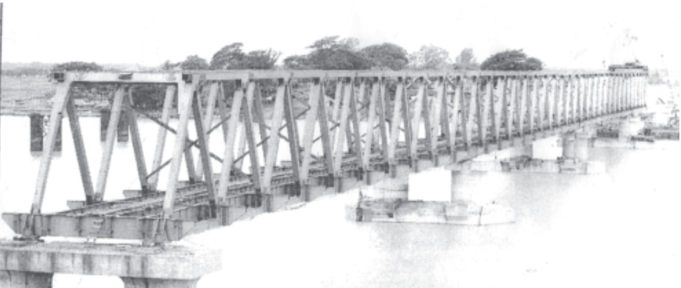
Progress in construction of Sittoung Bridge (Moplin). — MNA
