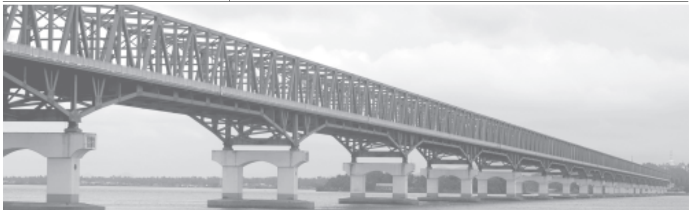
The magnificent Thanlwin River Bridge (Mawlamyine), the longest in Myanmar. —MNA
