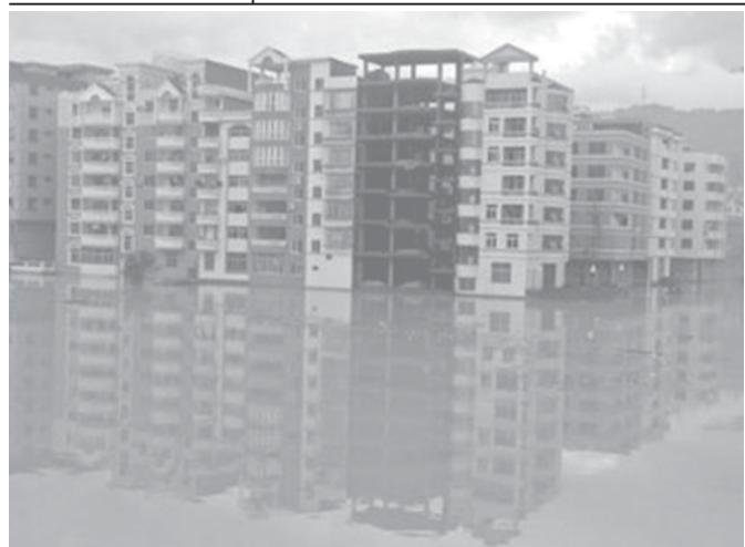
Residential buildings are flooded in Minqing County, east China's Fujian Province on 7 June, 2006. —INTERNET
