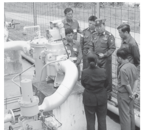
Minister for Energy Brig-Gen Lun Thi visits Mann Thambayakan refinery in Minhla Township, Magway Division. — ENERGY
