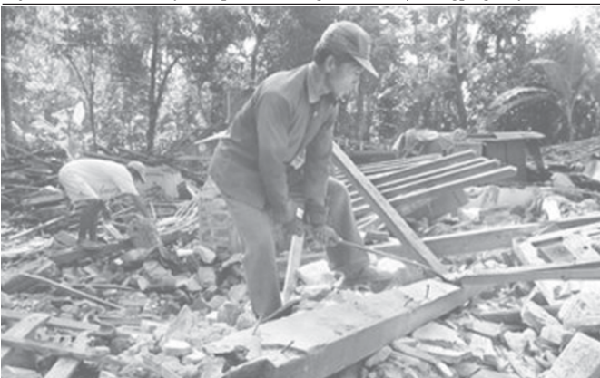
Residents clean up debris at the ruins of a house in Bantul, Indonesia, on 5 June, 2006. A 6.3-magnitude quake struck the region on 27 May, killing at least 5,782 people and damaging more than 130,000 homes, government officials said.—INTERNET
