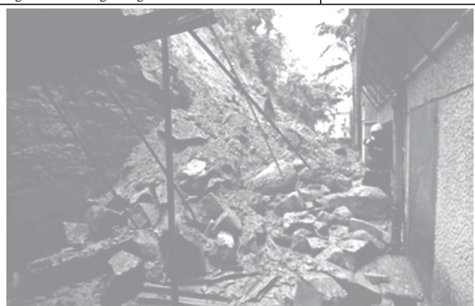
A rescuer works at a site of landslide, caused by continuous heavy rain, next to a dormitory near Fuzhou University, east China's Fujian Province on 1 June, 2006. About 200 people were evacuated immediately from the spot, China Daily reported. —INTERNET
