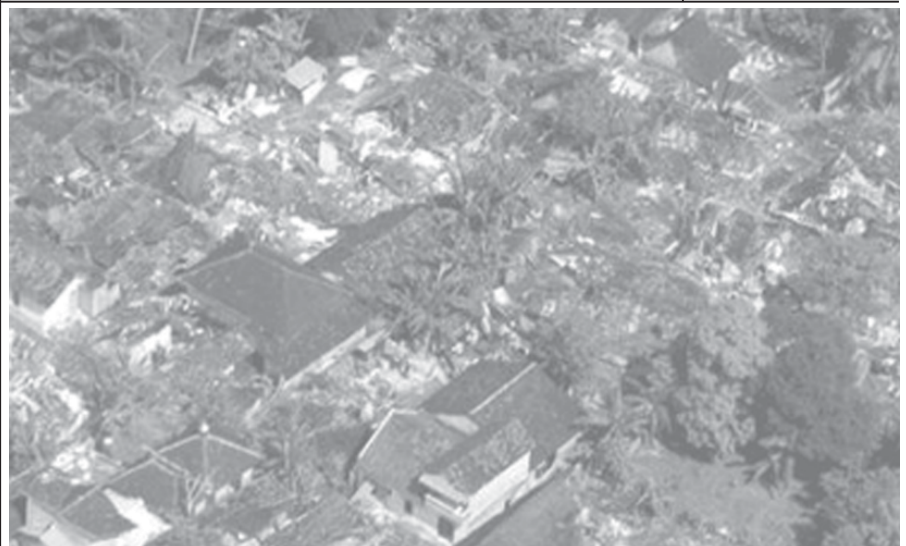
An aerial view of damaged houses in Indonesia's Bantul District, on 29 May, 2006.—INTERNET
