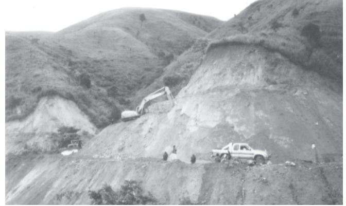
A section of Kengtung-Mongpyin-Tarkaw new road.
