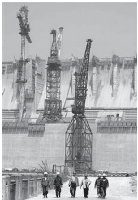
Workers walk in front of the Three Gorges Dam on the Yangtze river in central China's Hubei Province, on 17 May, 2006.
