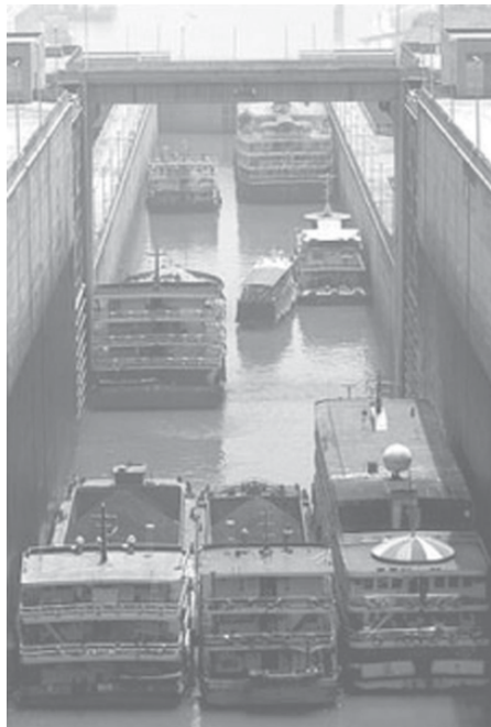
Ships travelling upstream on the Yangtze River pack into a ship lock at the Three Gorges Dam project in Yichang on 17 May 2006. After 13 years of immense physical effort and technical ingenuity, China put the finishing touches to its controversial Three Gorges Dam, the world's largest hydropower project.
