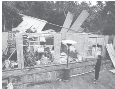
A woman looks at the damage after strong winds from Typhoon Chanchu tore the roof of a storage area in Hong Kong. Almost 300 Vietnamese fishermen remain missing and 28 have been reported dead, three days after Typhoon Chanchu sank at least 11 ships in the South China Sea. — INTERNET
